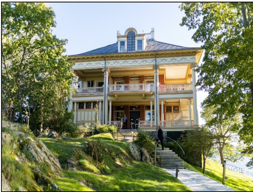
The approach to the beautifully maintained historic clubhouse today. During the heyday of rail travel Squantum was important enough to have their own station
