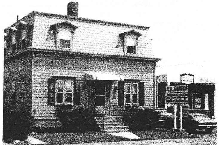
INGRAHAM'S CORNERS , the intersection of Warren Ave. and Broadway was named for the builders of this Victorian Italianate style home. The town jail was once housed in the basement.
