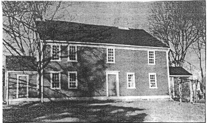
THE PHILIP WALKER HOUSE, 1676, is located at the corner of North Broadway and Massasoit Ave., Rumford. It is the oldest house in the area.
